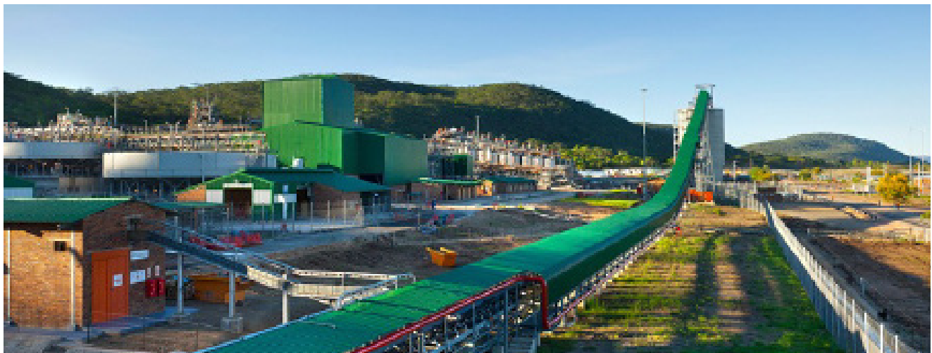
Unki Mine concentrator plant in Zimbabwe
